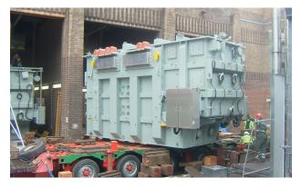
Although the Bankside Power Station ceased operation several decades ago, the substation continued to operate and remains an important part of London's electricity network. The £60 million refurbishment of the substation included many substation upgrades, 6 power transformers from Wilson Transformer Company in Australia and an engineered heat reclamation system that used the losses of the transformers to supplement the heating and hot water requirements of the adjacent Tate Modern.
